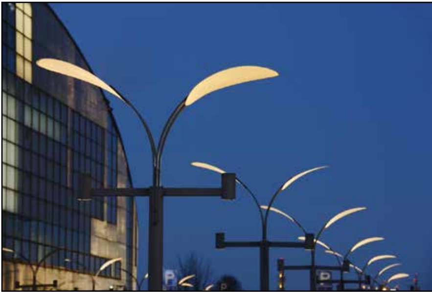
Transformation in distinct operational areas such as public safety, transportation or street lighting is multi-faceted
